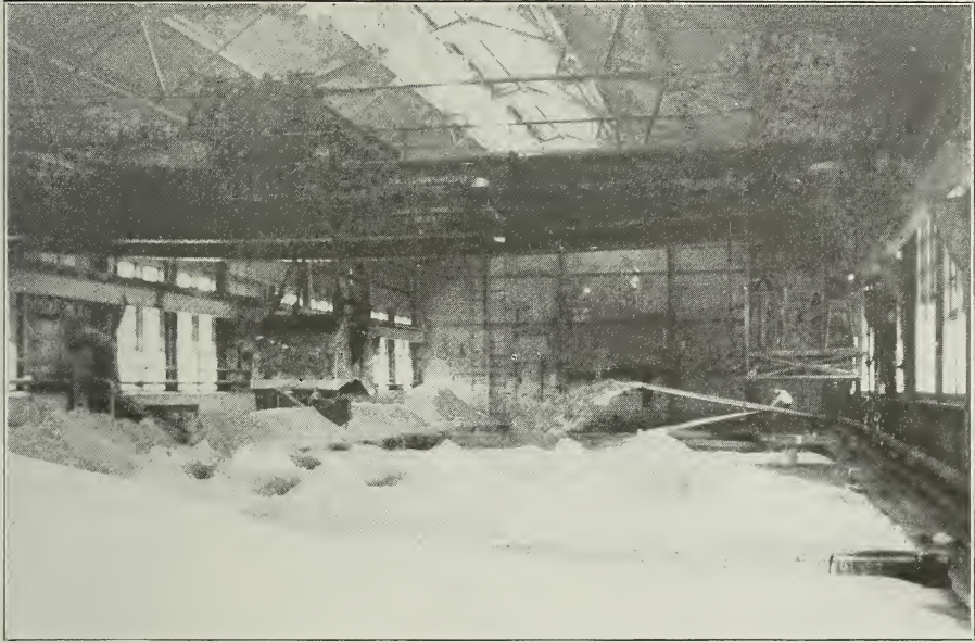
Fig. 27. Draining bins of Ottawa Silica Company. The sand is pumped from the washers into the bins and may be seen spraying out from the pipe at the right. The overhead crane removes the sand from the bins to the driers beneath the ridge of sand along the left wall of the building. (Photograph by courtesy of Ottawa Silica Company.)
